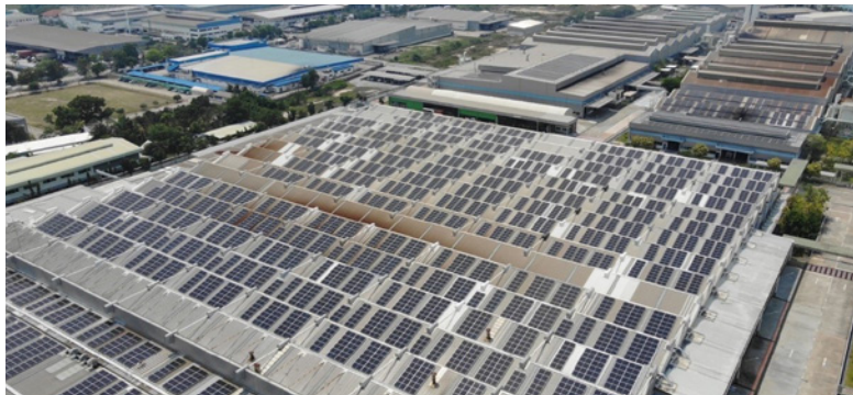
Solar panels introduced at STM
