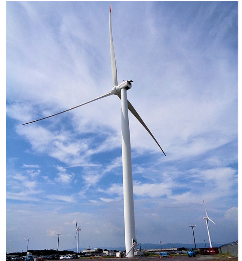
Wind power generator under construction at Tahara Plant
